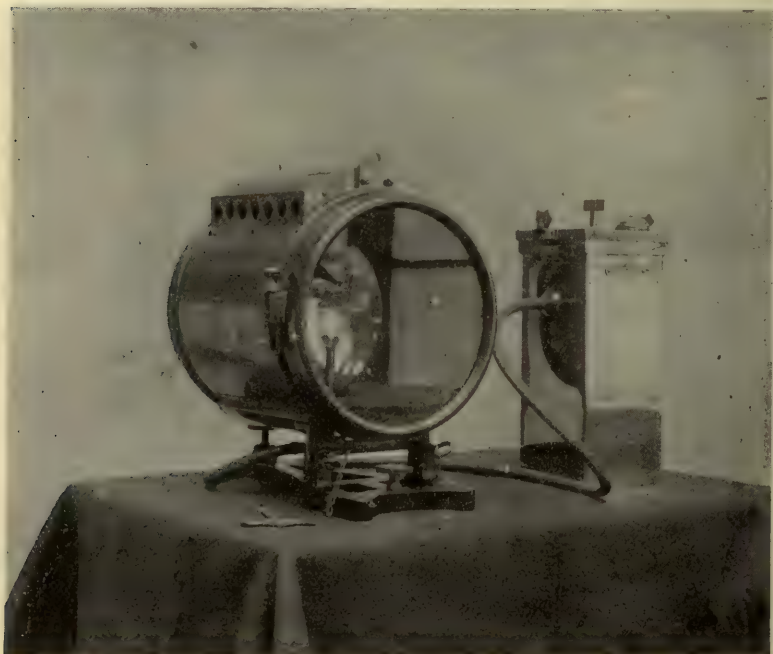
FIG. 15. Acetylene Signal Lamp. (Coast and Geodetic Survey.)
